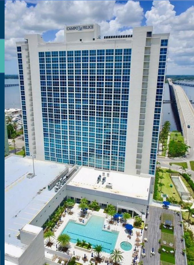
Hotel conversion in Fort Myers, Florida
